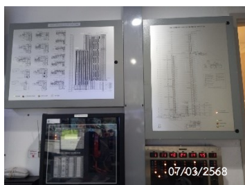
Graphic Annunciator Fire Alarm System
