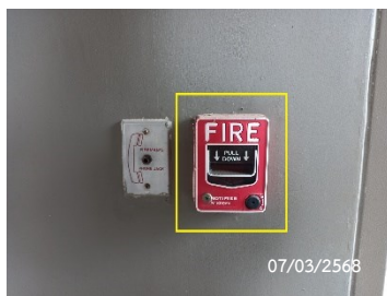
Fire Alarm Manual Station
